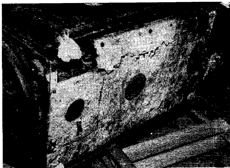
The crumbling base.
