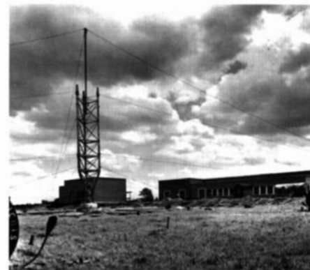
May 1949, mast under construction
