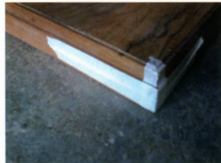
Repaired corner joint
