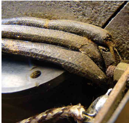
The original mains transformer voltage panel
