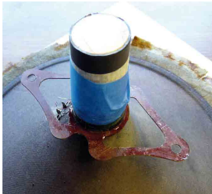
7: New coil in position
