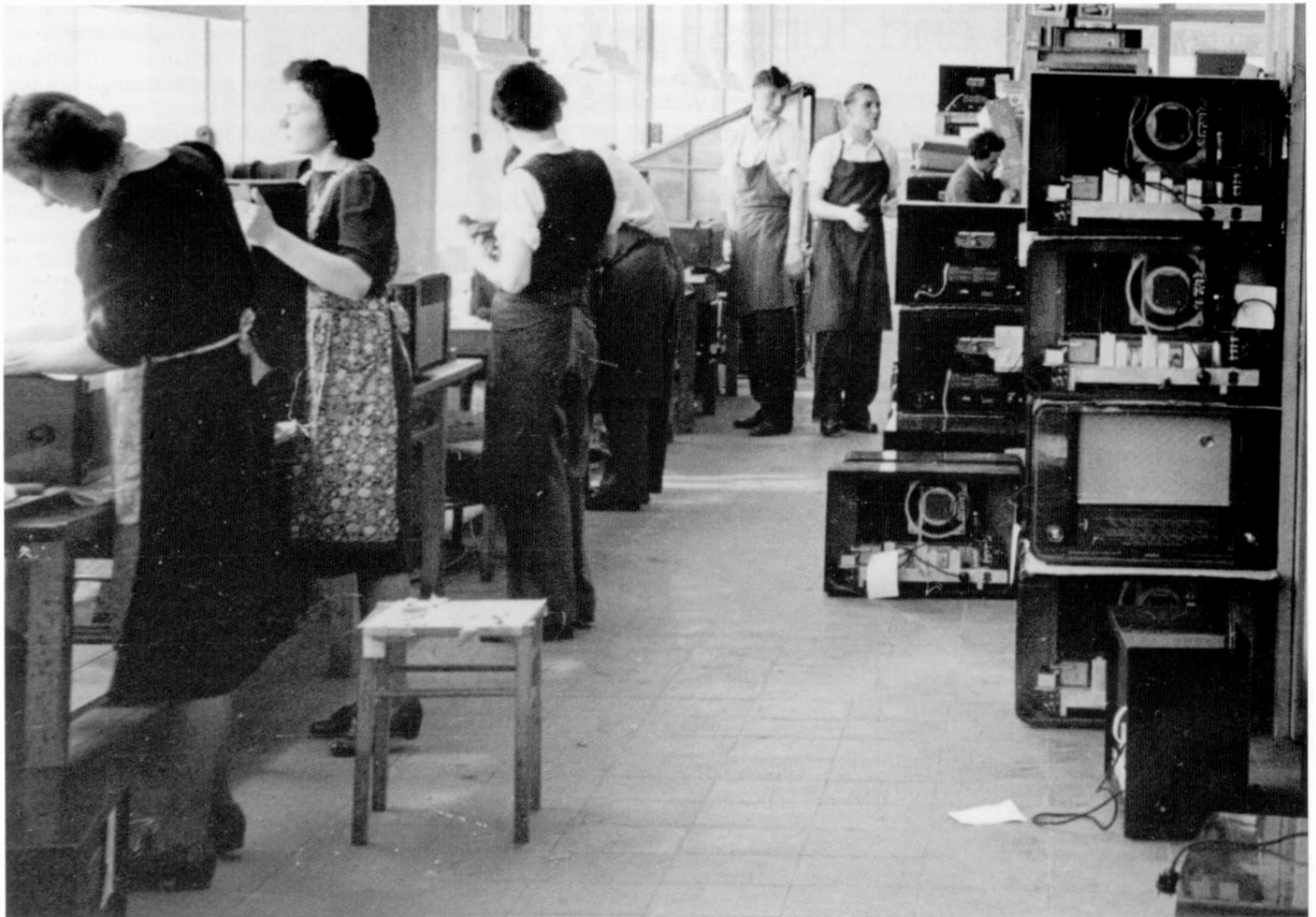
Repairs an final polishing at the Schaub and Lorenz works
