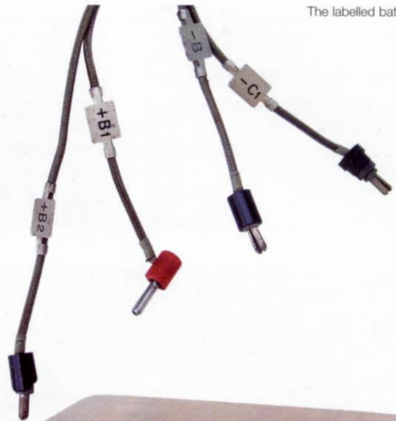
The labelled battery leads
