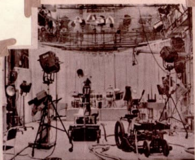
DISMANTLED AT LUNCH-TIME, the studio can now be seen with its remarkable collection of apparatus. The powerful array of large cameras up to 40 kilowatts when strong lighting is wanted. Note the main-line coils of arranged cables conveying the light impulses to the control room. There are two studios at the Alexander Palace.
