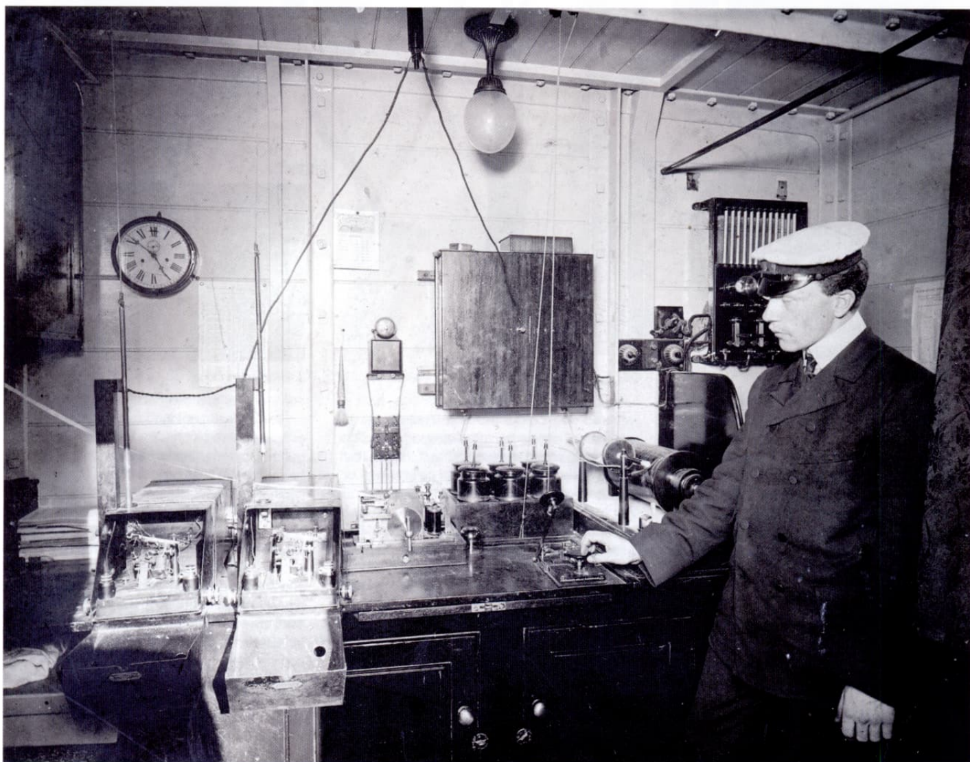
1. Interior of the wireless telegraph cabin on the SS Minnetonka , August 1904. (Reproduced from an original photograph probably taken for Marconi's Wireless Telegraph Co Ltd and held by the Science Museum, London. Science Museum Photographic Studio, image number B500092.)
