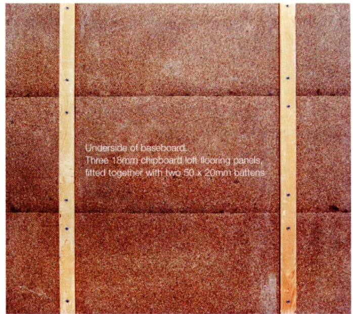
Fig 4: Underside of baseboard
