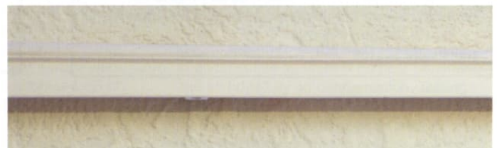
Big loop top pipe to run above the picture rail
