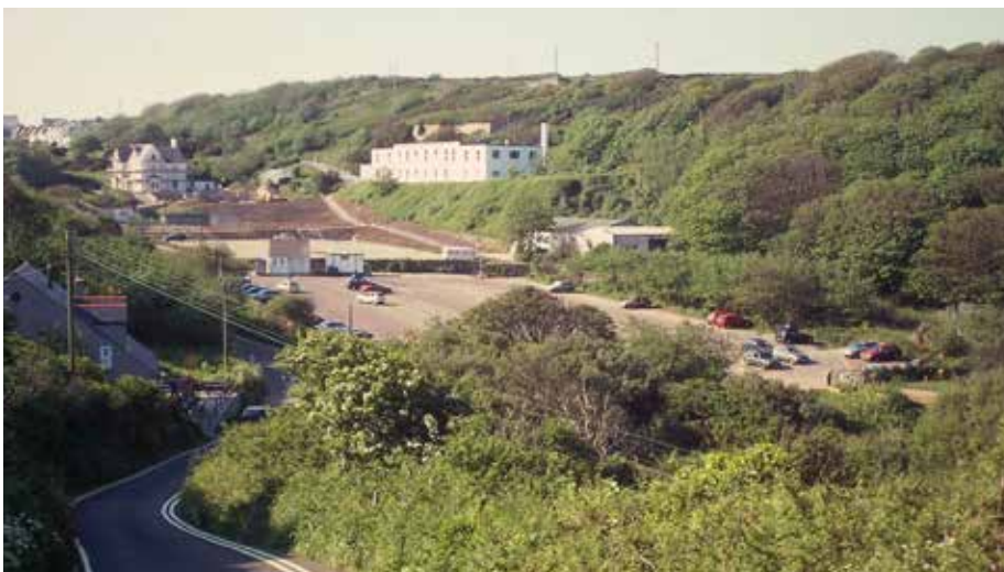
Fig. 2 Cable station from 1904-41 (centre) now housing archives and tunnel entrances with museum behind
