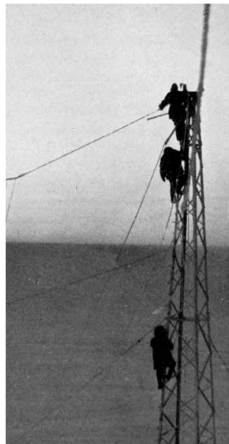
Figure 8 Climbing one of the radio masts at Little America 19 .
