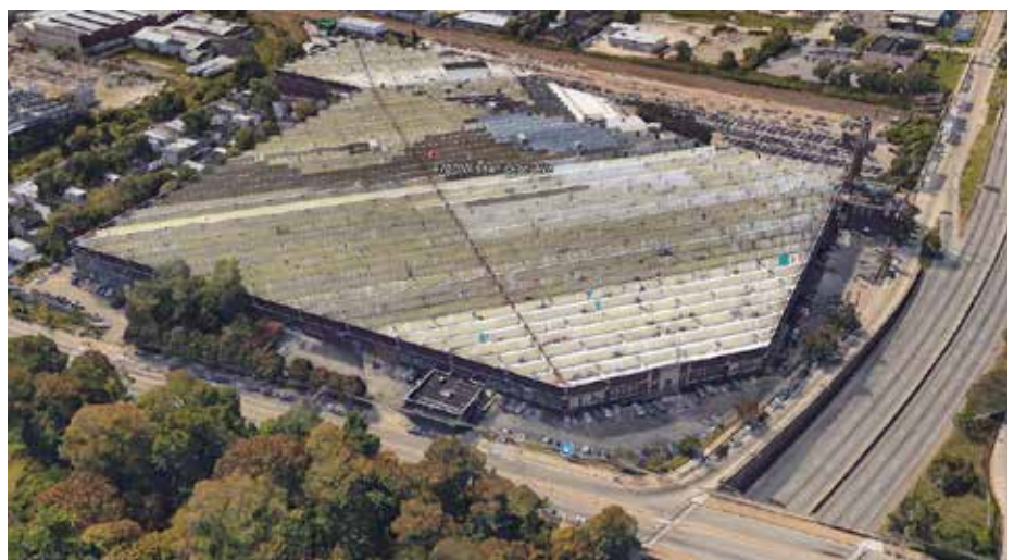
Figure 11 The 94 year old Atwater Kent 1924 factory today, courtesy of Google Earth. Like his products, Atwater Kent's factory was built to last. The building hasn't changed much in 94 years, but Philadelphia certainly has!
